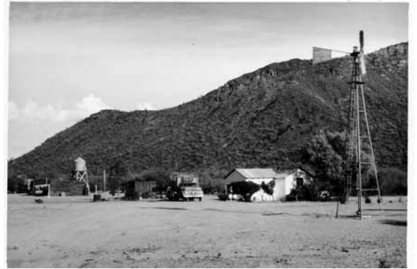
After Henry D. Gray bought the ranch, it continued as a working ranch until 1976. This is how it looked in its later days.
